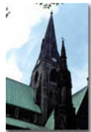
Tower at crossing
