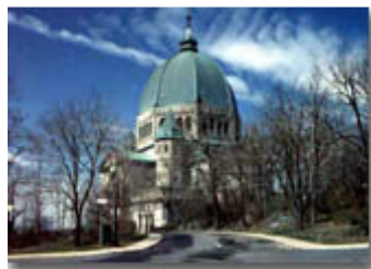
Exterior view Photo : François Brault
