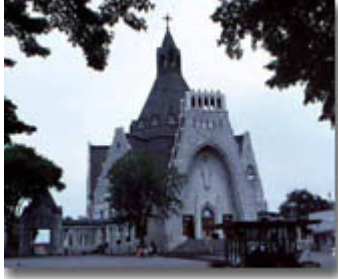
Exterior view of the new basilica Photo : François Brault
